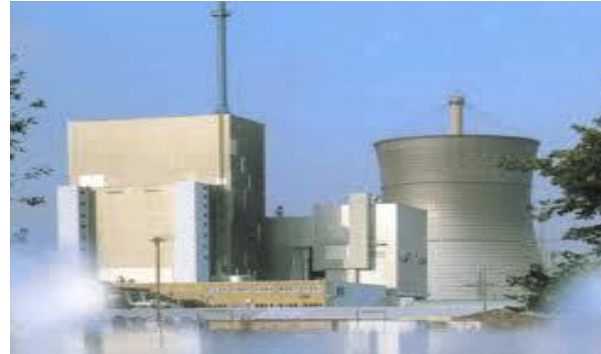
THTR, Germany 300 MWe 1986-89
