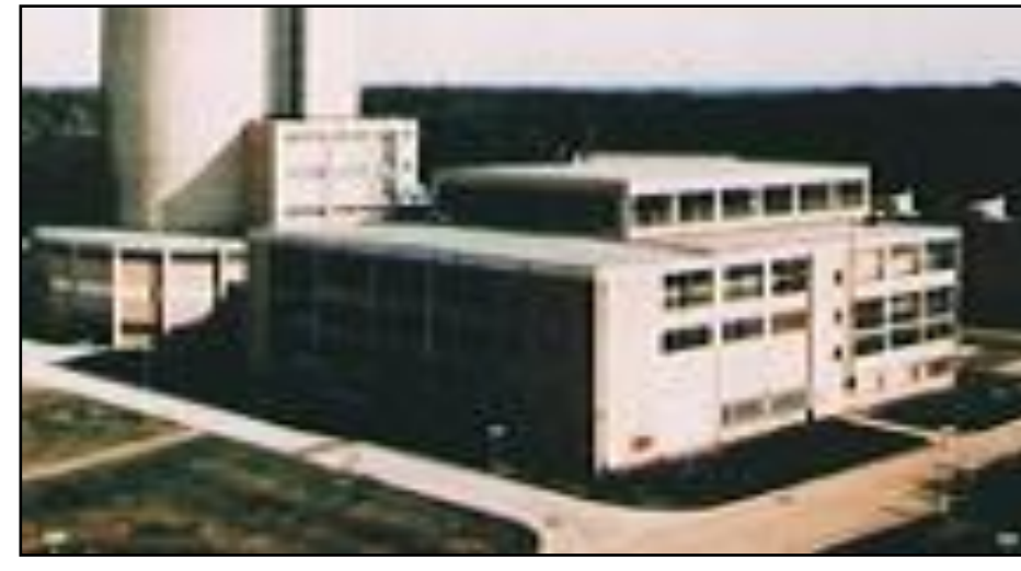
AVR, Germany 15 MWe 1967-88
