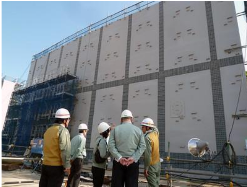
Construction 18m embankment to protect against tsunami Hamaoka NPP, Japan
